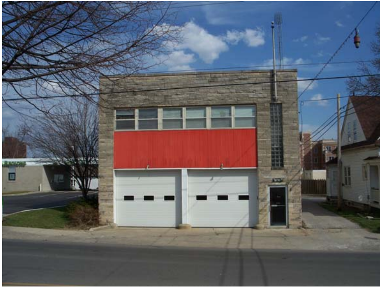
Rogers Street Firehouse, 105 S. Rogers Street
