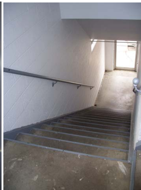
Stairwell & upper landing
